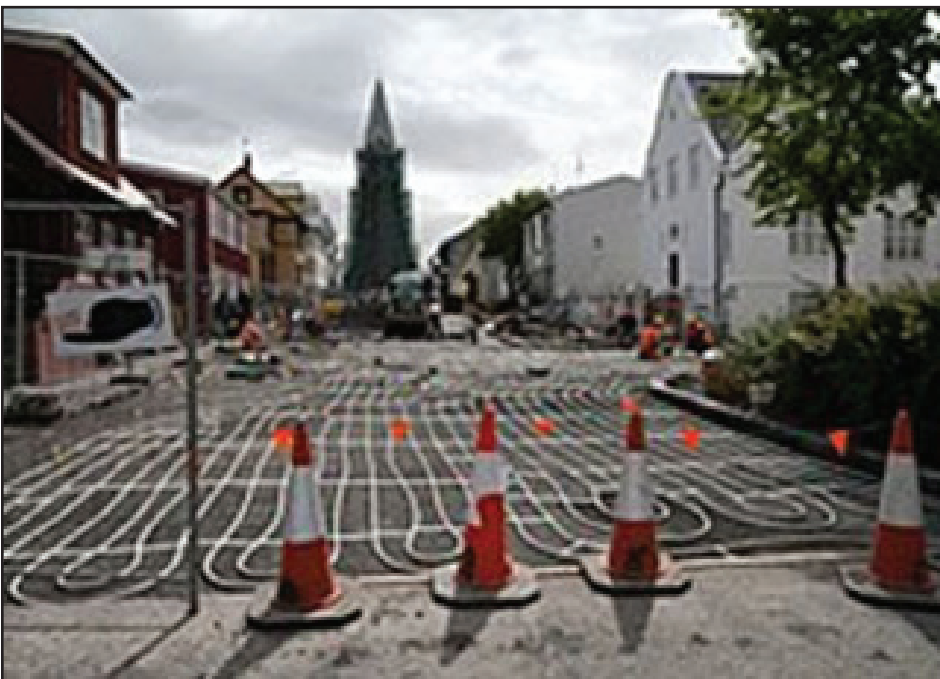
Pipes being installed under a road surface
